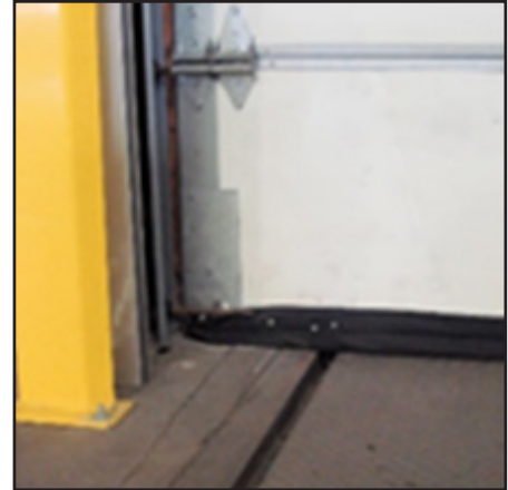
Example of bottom edge door seal
