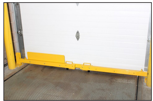
Example of protective barriers installed to protect door tracks
