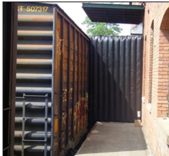
Metal hoods over dock door, railcar door, and MRI inflatable seal
